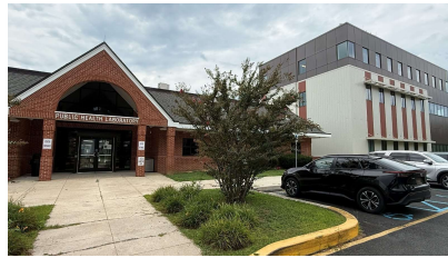
Delaware Public Health Laboratory Three-story addition totaling 70,816 sq. ft., with site, building, fire alarm, and fire suppression system permits.
